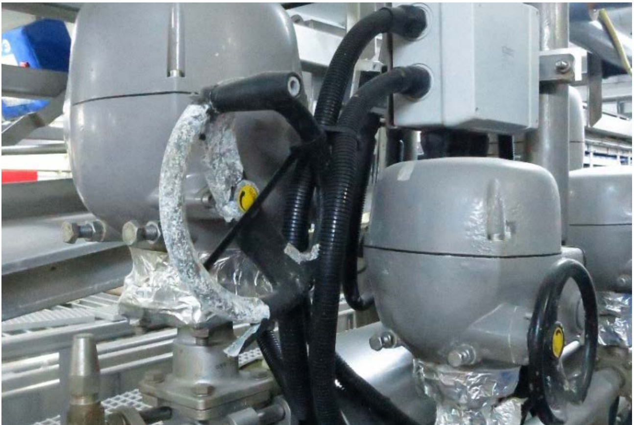
Figur 4-13 Malt ventilhjul i aluminium
