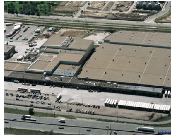
Safeway distribution terminal
